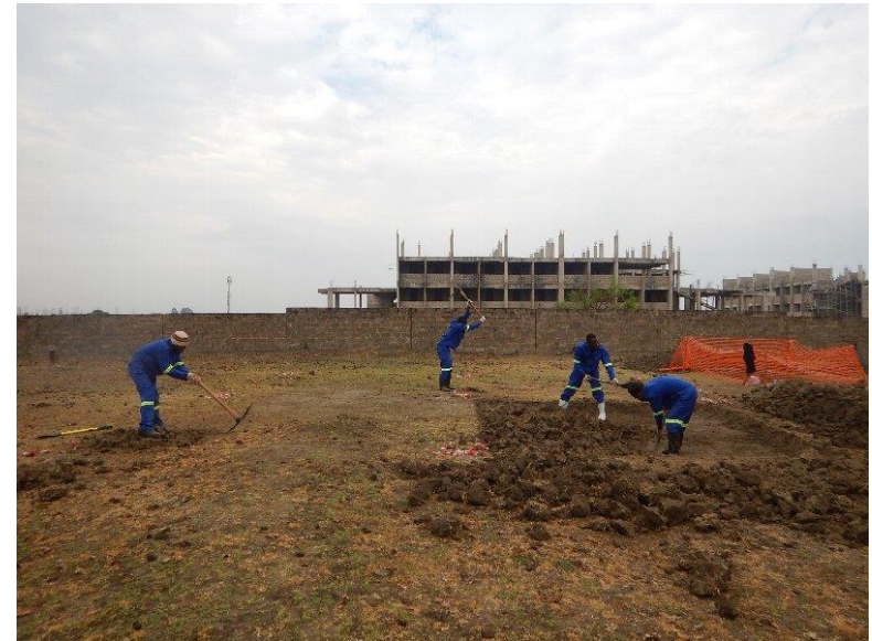
Excavation of surface soil for pilot tests
