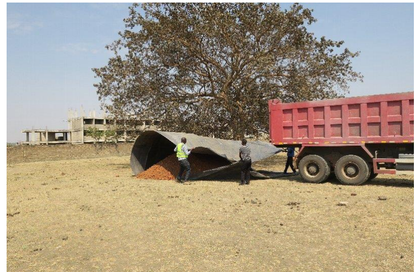
An impermeable sheet is used for storage
